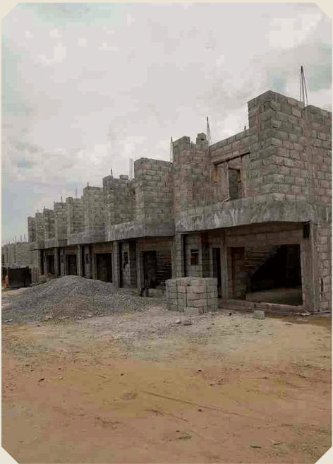
RECORD II · BLOCKWORK
